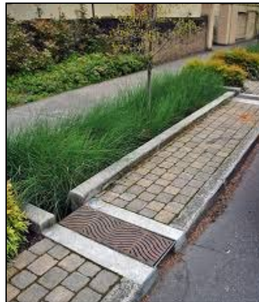
Roadside bioretention. Source: sitephocus.com
