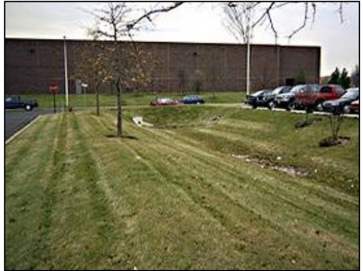
Grassed swale. Photo Source: EPA
